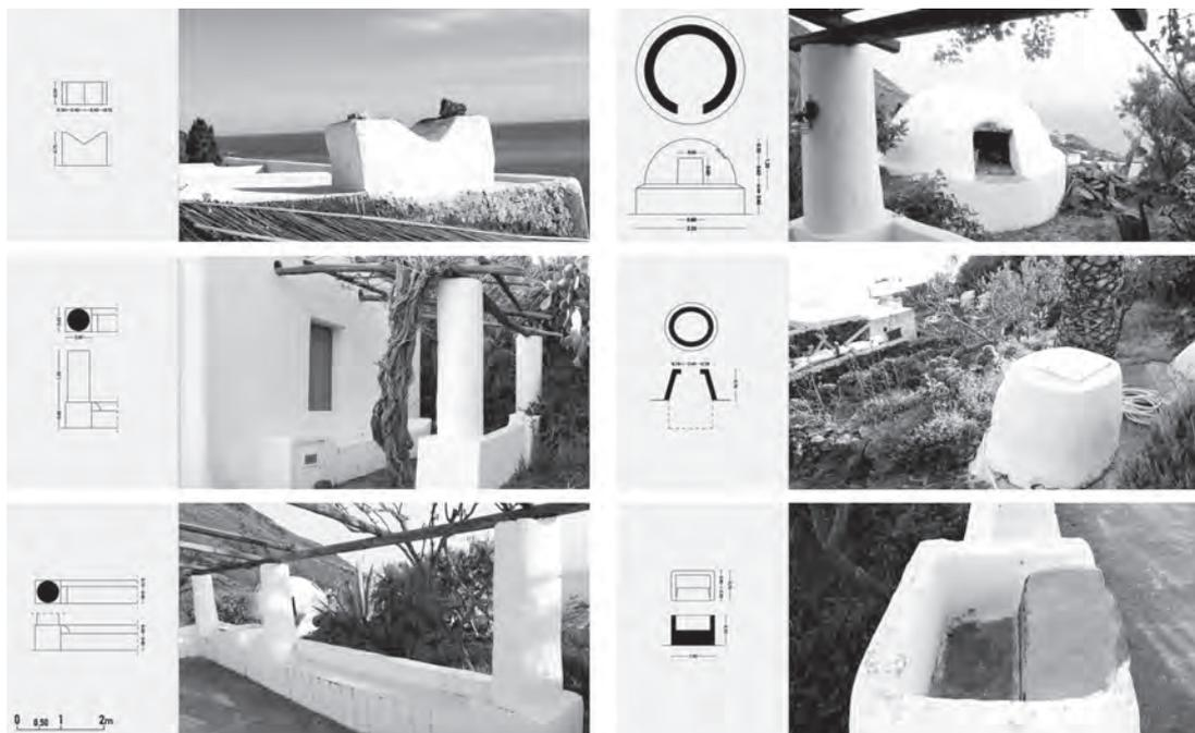
[5] The service elements of the home: roof battlements (“*pizzi*”), oven (“*fùrnu*”), column (“*pulèra*”), underground cistern (“*jistèrna*”), stone bench (“*bisòla*”) and waterbasin (“*pila*”).
